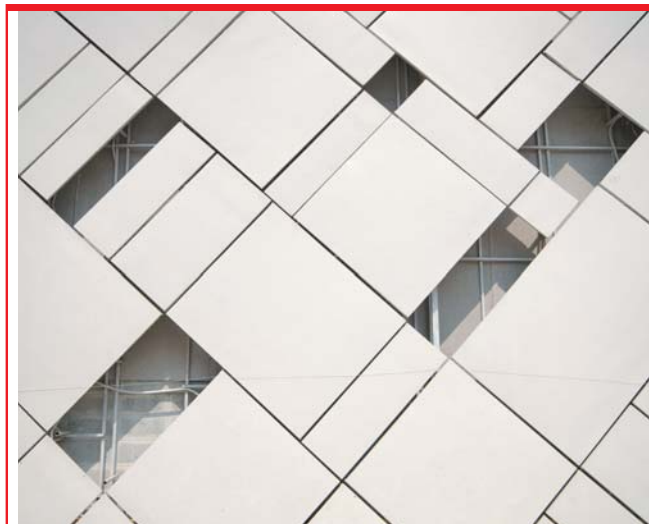
External Wall Creating space lining by using SCG SmartBOARD Squared Edge 8 mm. thick
