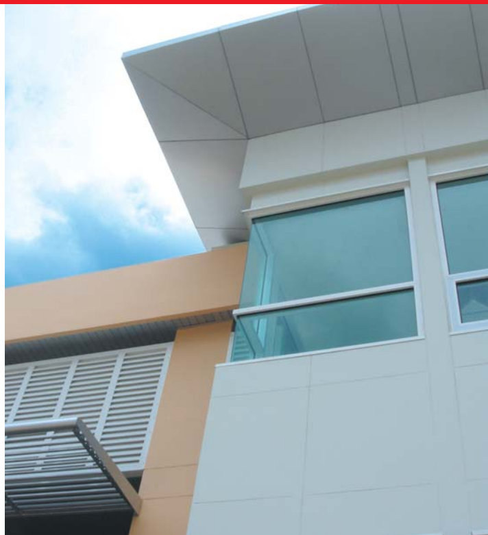
External Cladding Metro Park Condominiumtown, Bangkok
