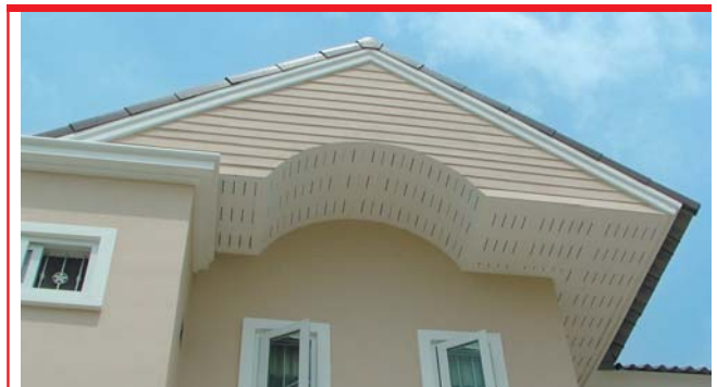
External Ceiling Using SCG SmartBOARD Ventilated Wood Grain 4 mm. thick.
