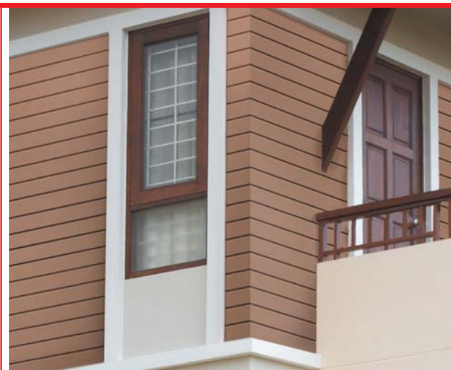
External Wall Using SCG SmartBOARD 4 inch Lining 8 mm. thick.
