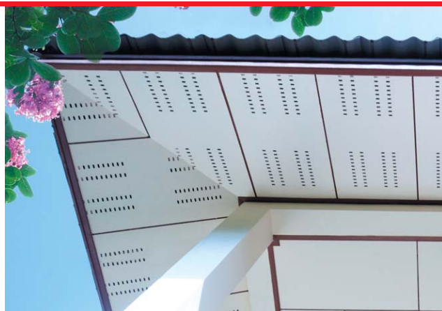
External Ceiling Using SCG SmartBOARD Ventilated 4 mm. thick.
