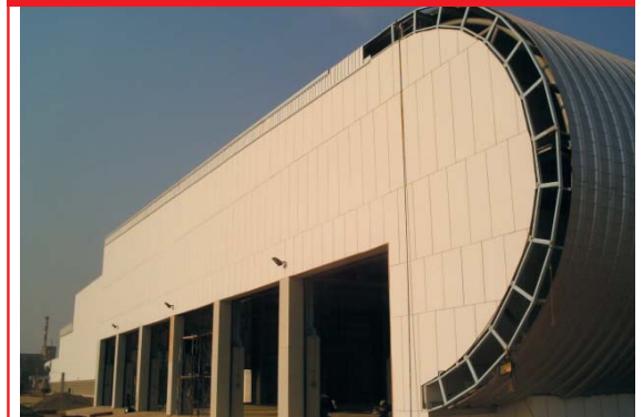
External Cladding Phenix pulp and paper plant, Khonkaen
